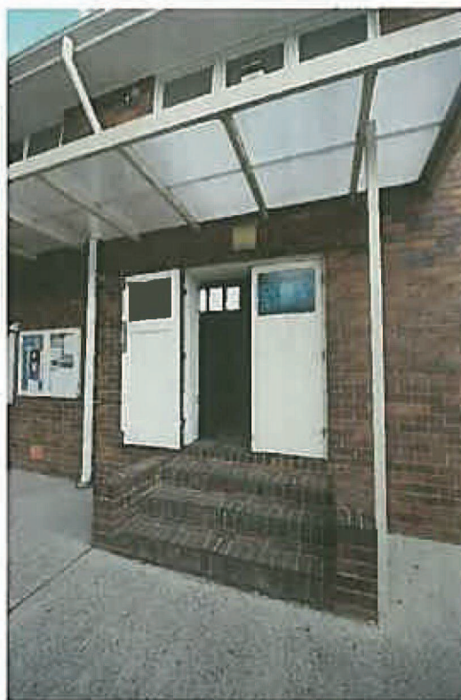
Figure 39: Detail of northern doors to Gymnasium, with modern awning above.
