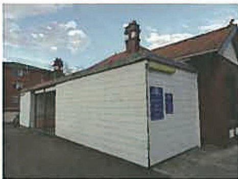
Figure 42: West elevation of side verandah enclosure
