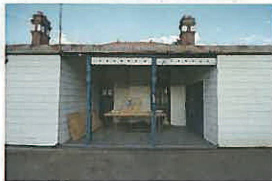
Figure 43: Detail, west elevation verandah, showing early timber posts and frieze in unenclosed section of the verandah
