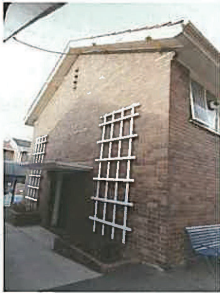
Figure 32: Western elevation, main entry to Ethel B Wallis Memorial Gymnasium
