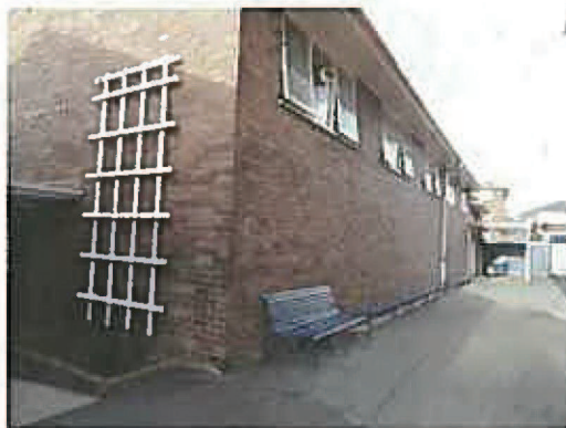
Figure 34: Southern elevation and part of western elevation, Ethel B Wallis Memorial Gymnasium
