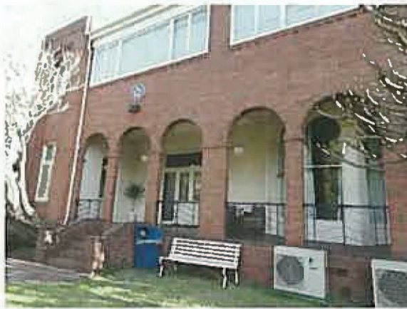
Figure 14: Detail, ground floor eastern end of north elevation, showing colonnade and details of The Briars including faceted bay window (at right)
