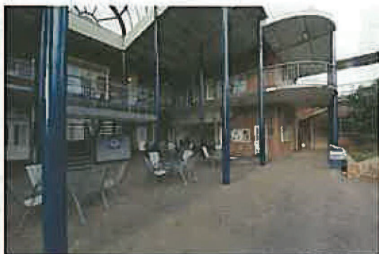
Figure 22: View of rear (southern) elevation of Wallis Hall, showing modern (1990s) additions
