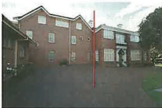
Figure 18: Eastern elevation of Wallis Hall. The red line marks the start of the 1990s rear extension.
