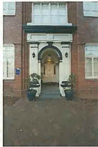
Figure 17: Detail of the eastern entry of Wallis Hall, part of The Briars
