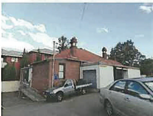
Figure 44: Rear view of Fairhaven, showing roller door at rear of west verandah enclosure, concrete ramp at rear
