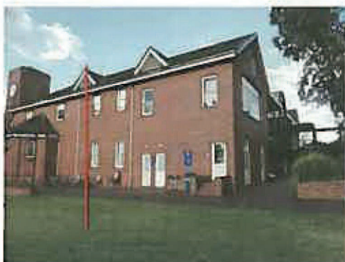
Figure 20: Detail, rear of western elevation of Wallis Hall. Red line indicates where rear additions begin. At the first floor level, there is a bricked-up window just left of the red line.
