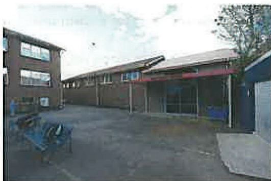
Figure 36: The southern elevation of the Gymnasium, with Pottery Room (7) and storeroom (19) at right
